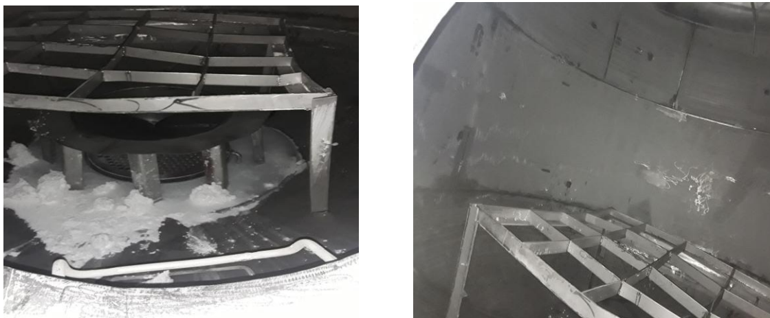
Figure 4 As found condition of S-402 after 1.5 years operation, with flushing practices
