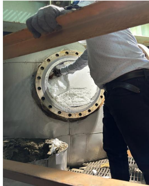
Figure 2: As found S-402 (heavily choked)
